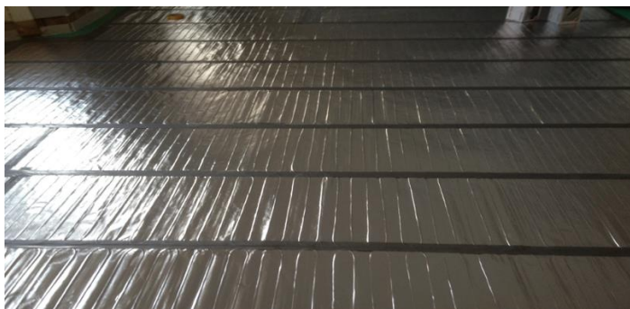
Fig. 10) Completed AluMat installation
