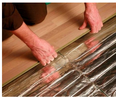
Fig. 11) Laying the wooden floor
